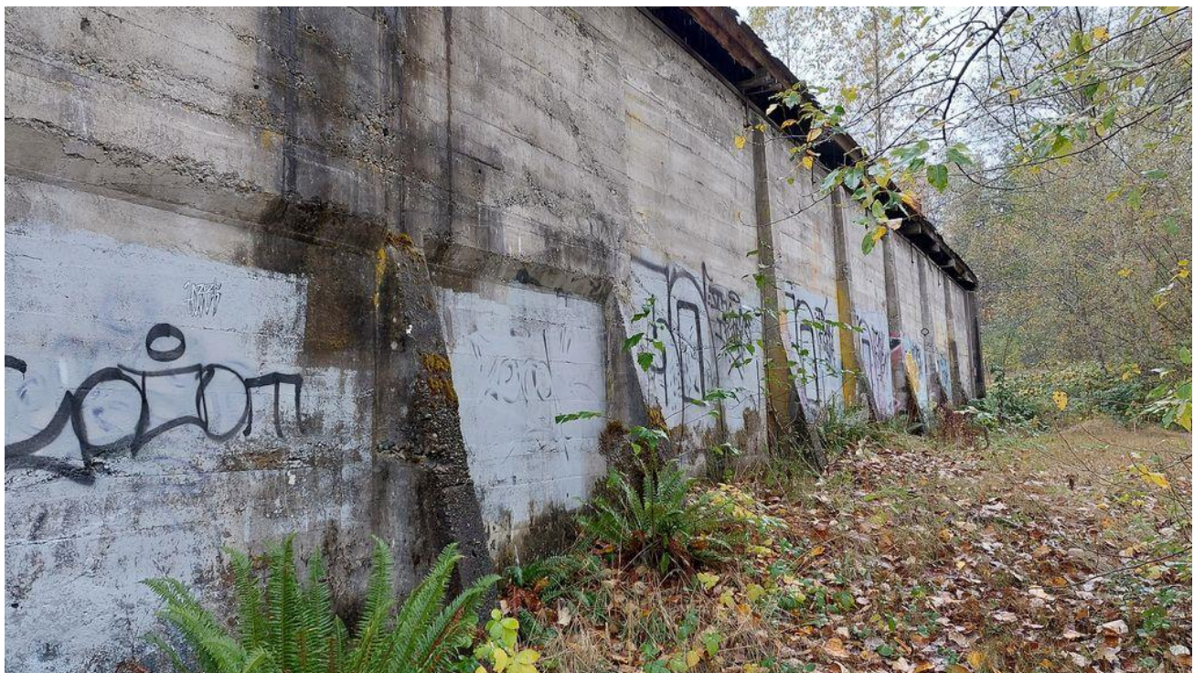
Figure B4. Concrete buttresses on north side, camera facing W
