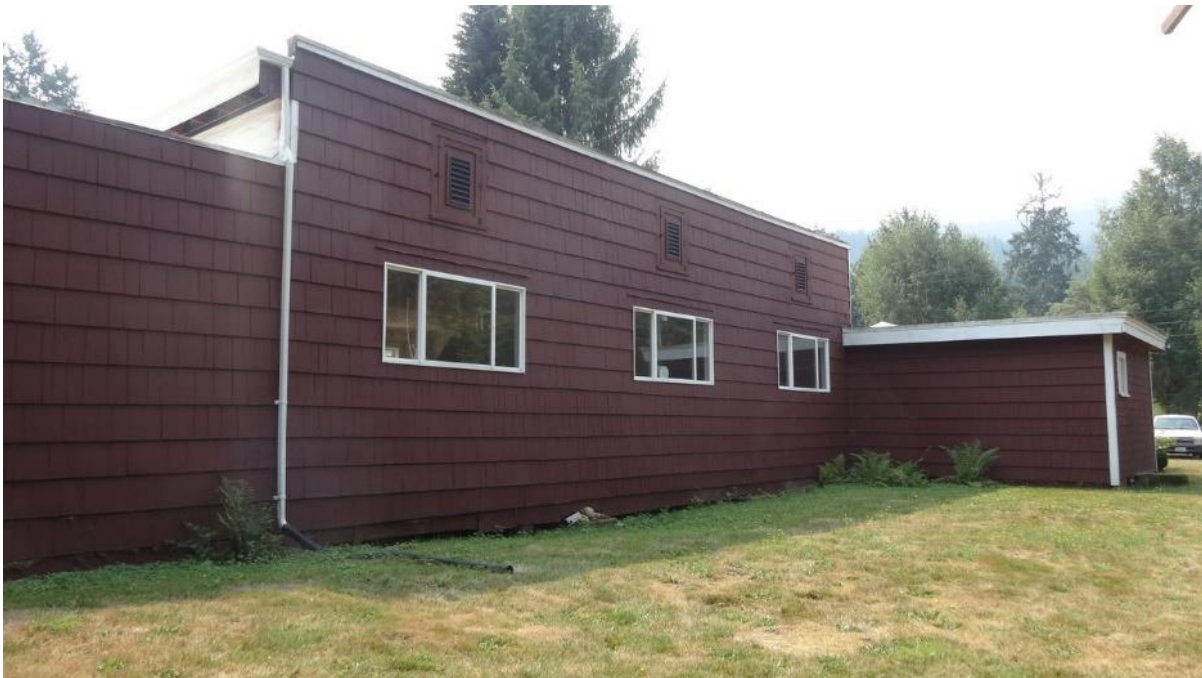
Figure C14. Vasa Hall's north side, view facing south. Note the three louvered shutters over clerestory openings that provide ventilation and access to the attic space, pictured above.
