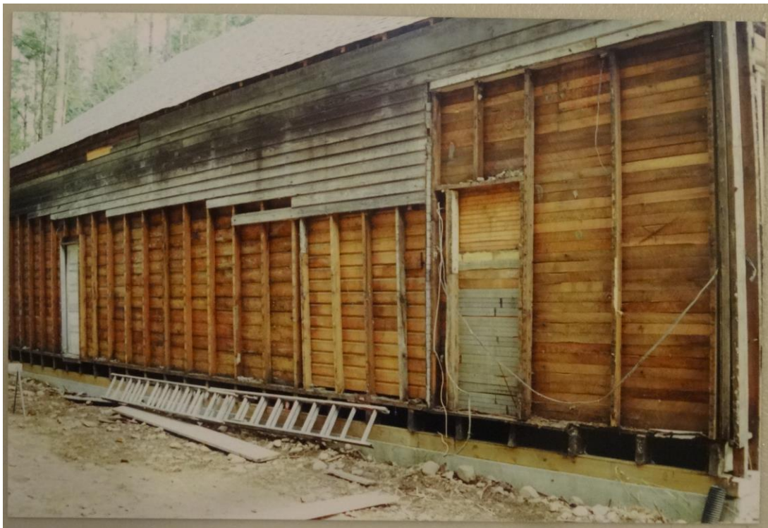
Figure B29. View of the west wall showing the consolidation and reuse of original materials during renovation, 1999-2000. Source: MVHS Scrapbook Coll.
