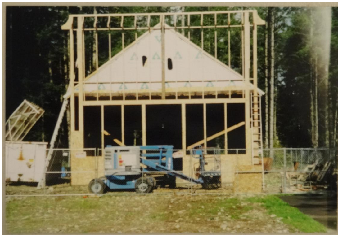
Figure B27. View of the new false front framing during renovation, 1999-2000. Source: MVHS Scrapbook Coll.
