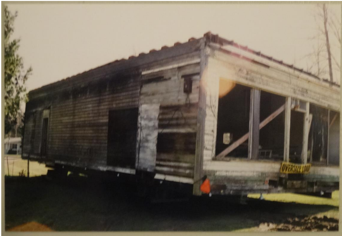
Figure B23. View of the rear side of the Gibbon General Store shown in its third location, with the false front and roof structure removed in preparation for relocation. 1999. Source: MVHS Scrapbook Coll.
