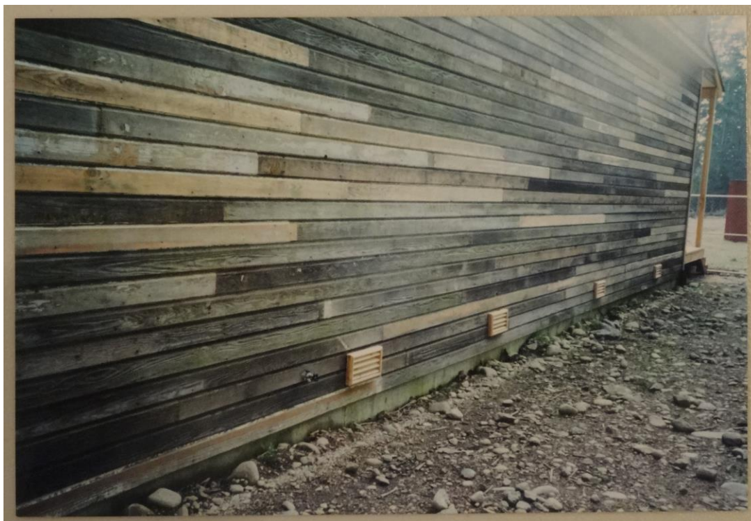
Figure B29. View of the west wall showing the consolidation and reuse of original materials during renovation, 1999-2000. Source: MVHS Scrapbook Coll.
