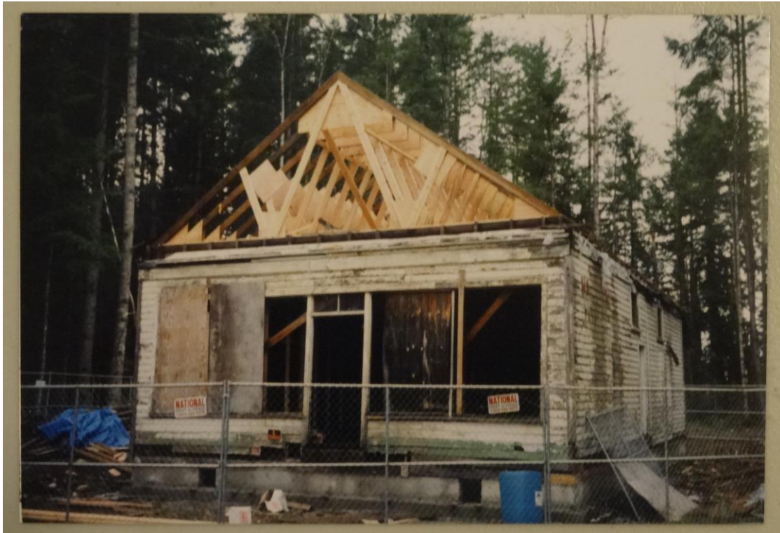
Figure B27. View of the new false front framing during renovation, 1999-2000. Source: MVHS Scrapbook Coll.
