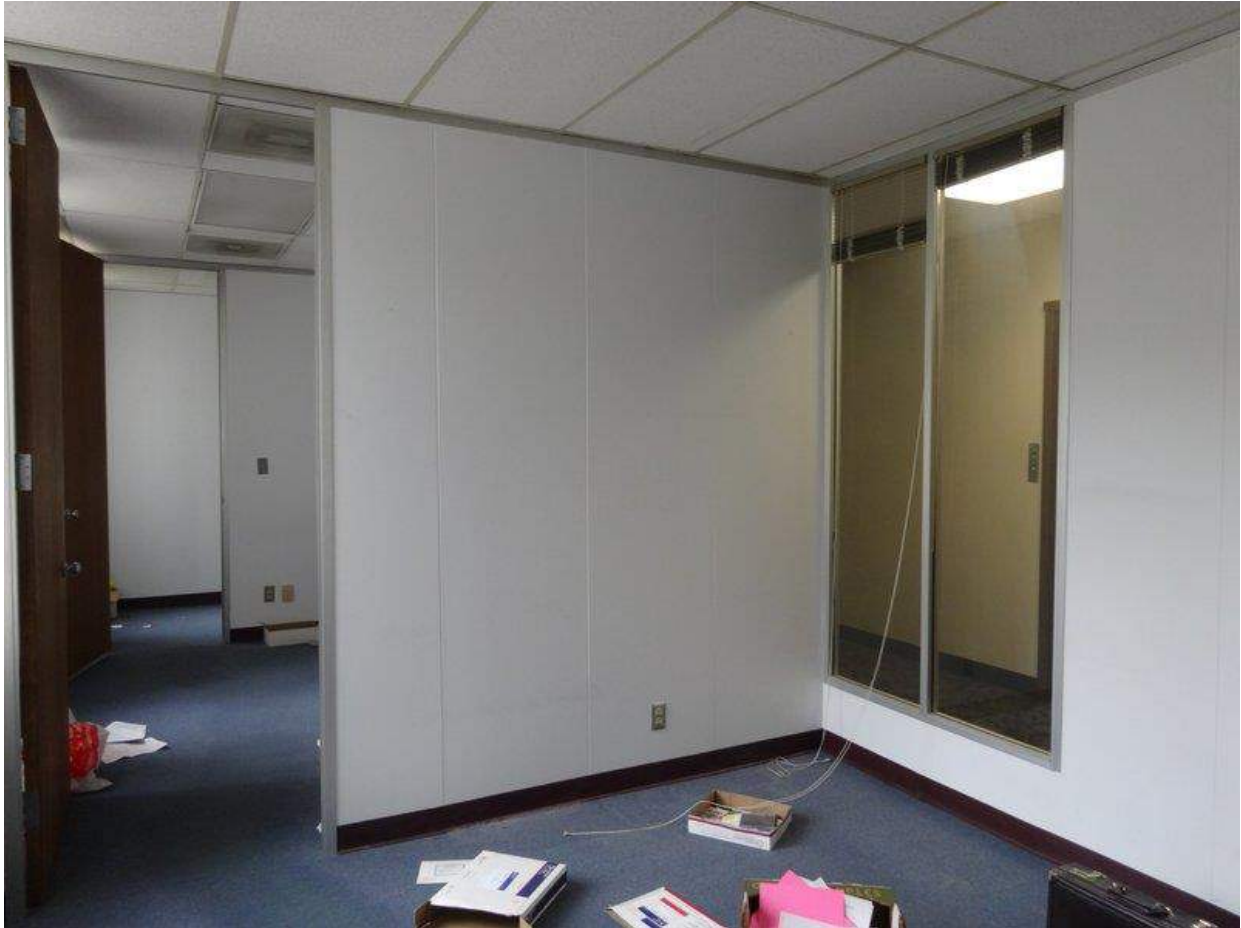
PHOTOGRAPH 42. Surrey Building, second floor. This is the suite of offices along the north side of the building. Note the metal door framing and scored walls, which are found throughout the second floor and appear to be original. The window looks into the hallway by the elevator. Camera facing southeast.
