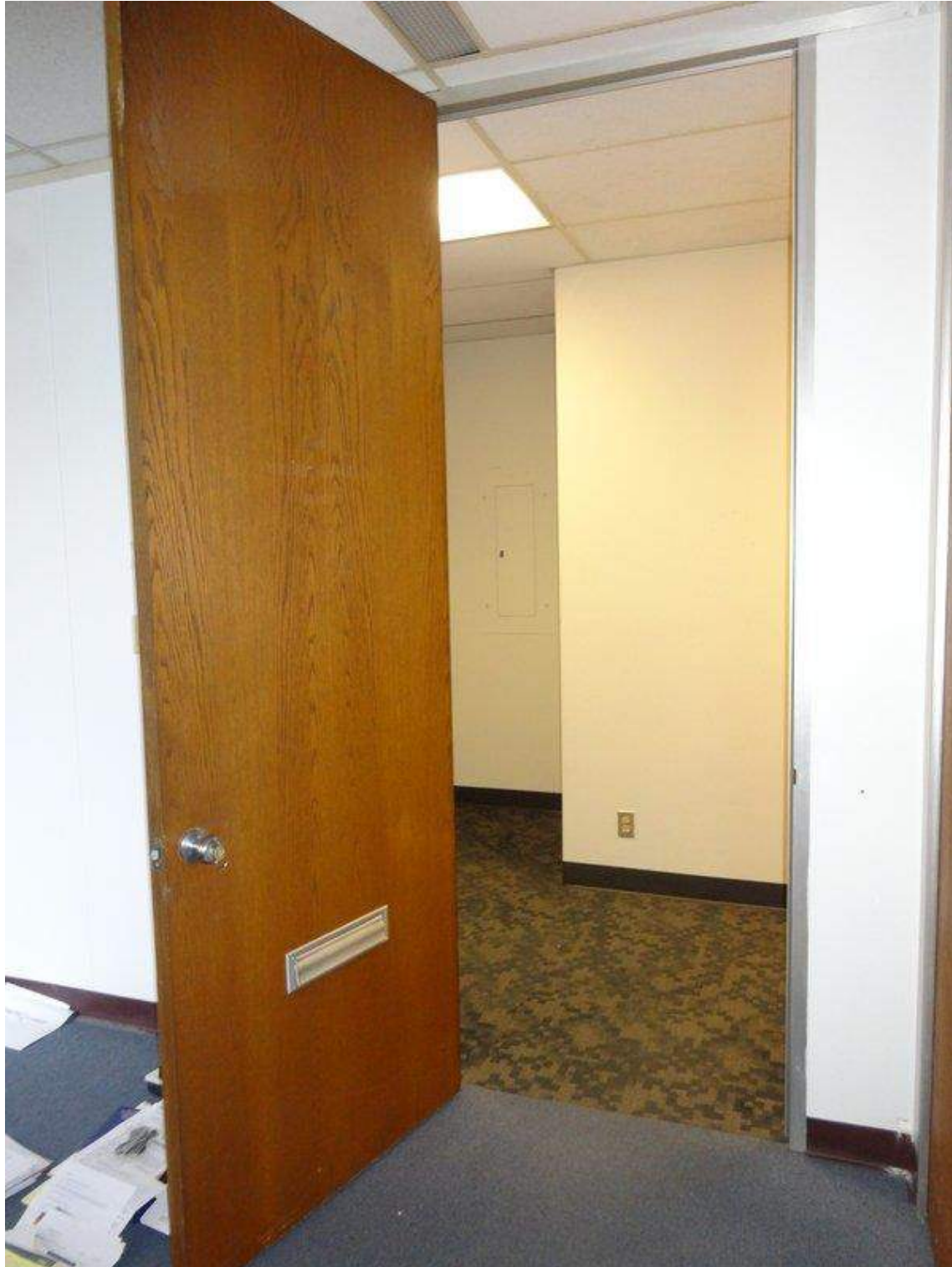
PHOTOGRAPH 41. Surrey Building, second floor. Entry into the office suite located along the north side of the building. This is a typical door, measuring 101" x 35", and has metal framing. Camera facing south.
